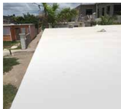
Finished roof with 3 coats of Sikalastic®-560.
