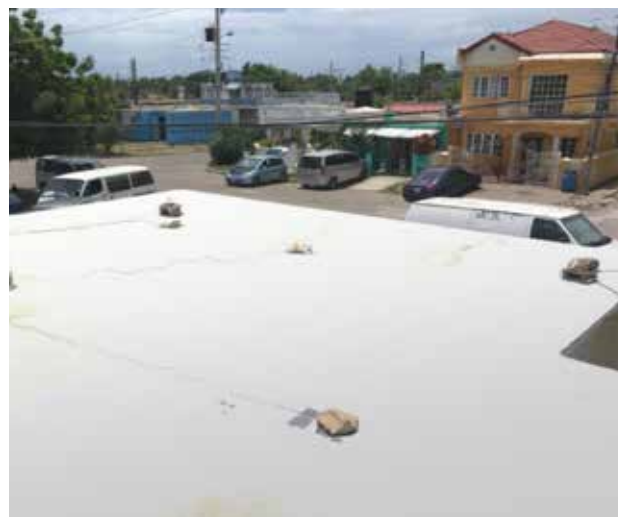
Roof after the application.
