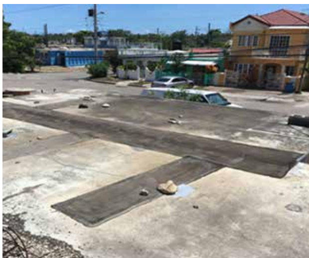
Roof before the application.
