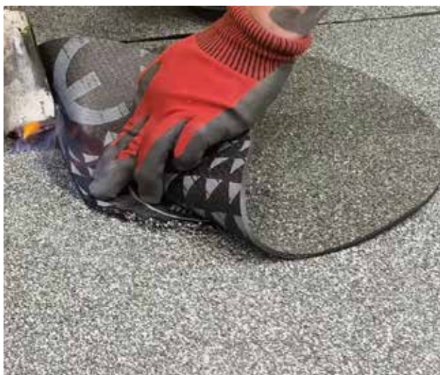
Torch application of the base sheet.
