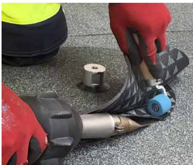
Hot-air application of the base sheet.
