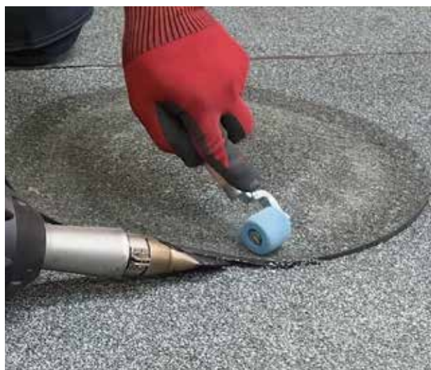
Hot-air application of the cap sheet.
