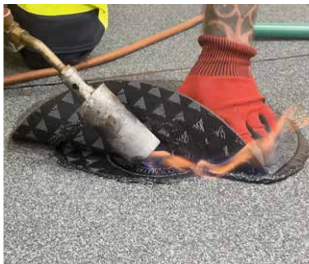
Torch application of the cap sheet.
