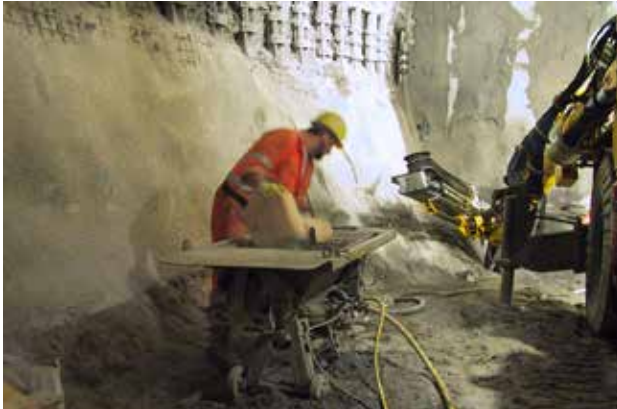
Temporary excavation stabilizing with dry sprayed mortar.
