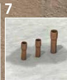
Leaking Penetrations i.e. Pipe Penetrations
