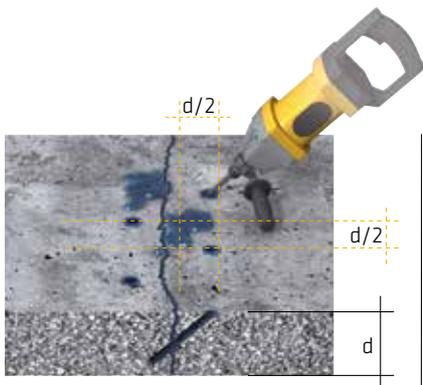
1. Drill holes for the packer alternating at a 45° angle to the concrete surface as shown in the picture.
