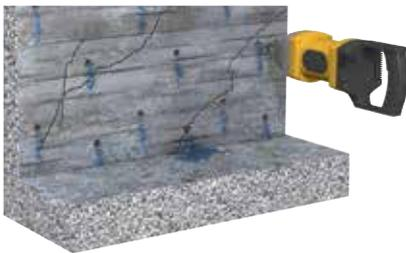
**1.** Drill holes for the mechanical packers through the leaking building component at a spacing of 30 - 50 cm as shown in the picture.
